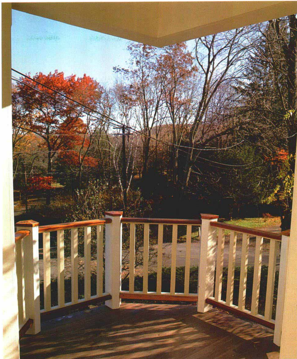
View from the octagon. The octagon's height and location make it a good lookout point, and the cable-tensioned handrail adds security. Above, the corner of the porch roof cantilevers over columns that frame the view. The decking is \frac{5}{4} Douglas fir finished with a clear deck stain.
